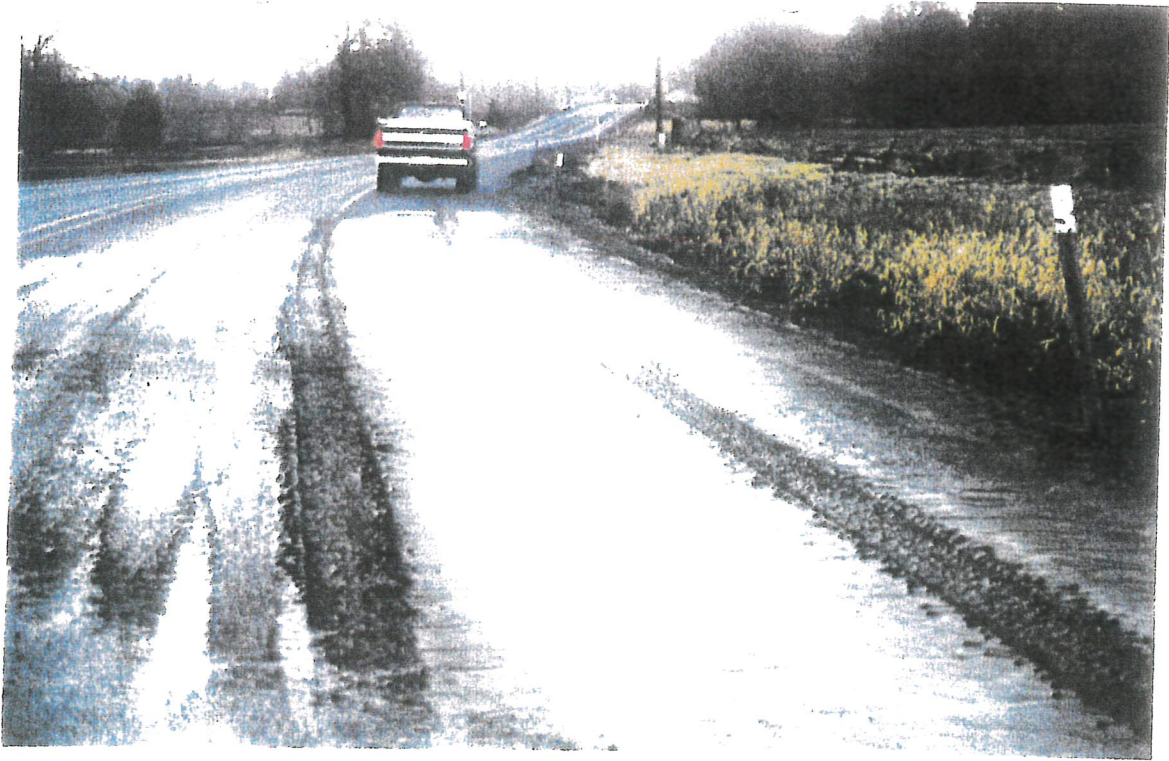
K. February 9, 1996 - 8:15 a.m. Looking south on Rush Road - mud on road after flood
