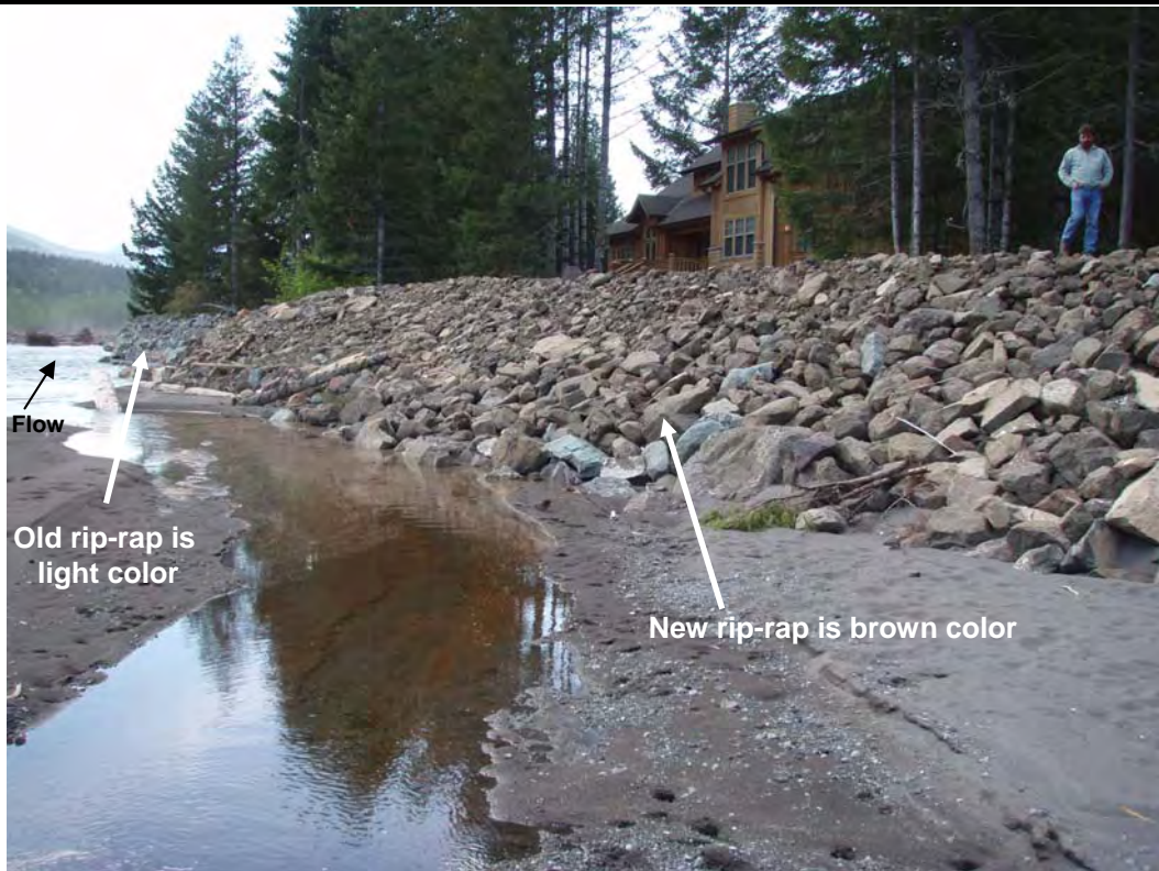
Photo 9: Facing south – New rip-rap placed in front of house in High Valley Community.
