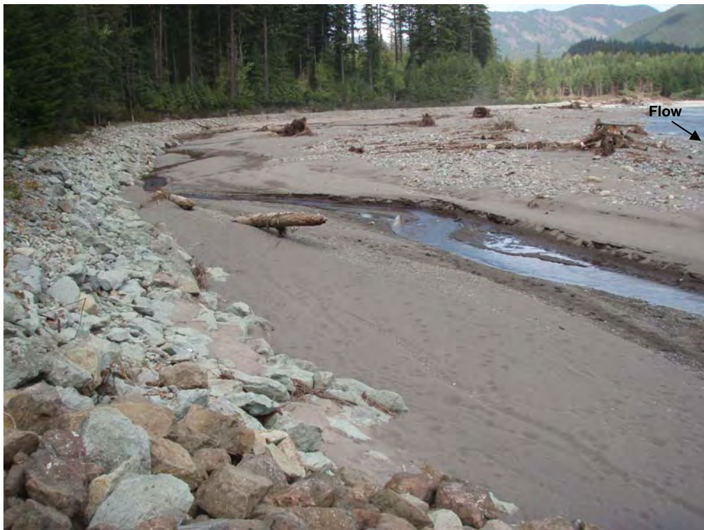
Photo 8: Facing north – Sand deposited against rip-rap on the right bank below the avulsion near High Valley community.
